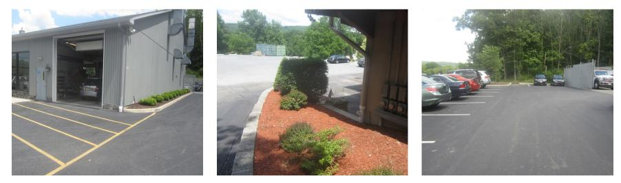
Stormwater is currently directed to the existing sewer system through connected downspouts. Parking spots can be replaced with porous asphalt to capture and infiltrate stormwater from the parking lot and roof. A cistern can be placed on the south corner of the building to capture roof runoff to be used for washing vehicles. A preliminary soil assessment suggests that more soil testing would be required before determining the soil's suitability for green infrastructure.
