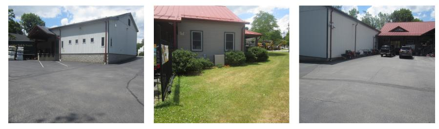
Stormwater is currently directed to the local sewer system by connected downspouts. A cistern can be installed on the south building to capture roof runoff. The water can then be used for washing vehicles or for other non-potable uses. A preliminary soil assessment suggests that the soils have suitable drainage characteristics for green infrastructure.
