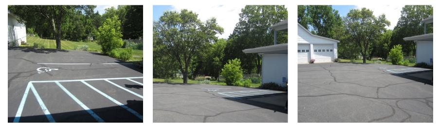
Stormwater currently flows across the parking lot. Parking spots adjacent to the south building can be replaced with porous asphalt to capture and infiltrate stormwater. A preliminary soil assessment suggests that the soils have suitable drainage characteristics for green infrastructure.
